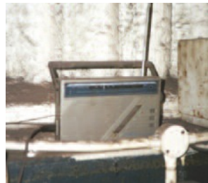
Sprayed coatings on wall
