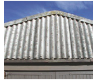
Asbestos cement panels
